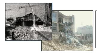
Failure caused by inadequate or no underpinning of the adjacent property
